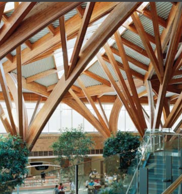
Carlo Fidani Peel Regional Cancer Centre, Mississauga, Ontario, Salter Farrow Pilon Architects
