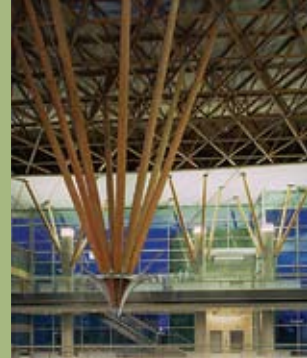
Thunder Bay Regional Health Sciences Centre, Thunder Bay, Ontario, Salter Farrow Pilon Architects
